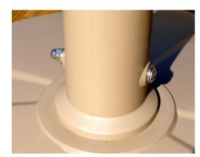
Remove umbrella pole and drill a 5/16" diameter clearance hole through each side of umbrella pole. Insert umbrella pole back in base and align holes with holes in center post. Insert bolt with 2 washers on each side and fasten nut as shown.
